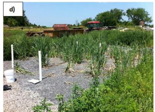
Wetland Construction: a) Pre-treatment tanks, b) Excavation with sand base, c) Placement of 30 mil liner, d) Installation of gravel and cattails.
